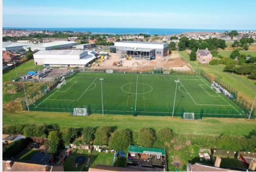
Berwick Sports and Leisure Centre works continue for completion in Summer 2023
